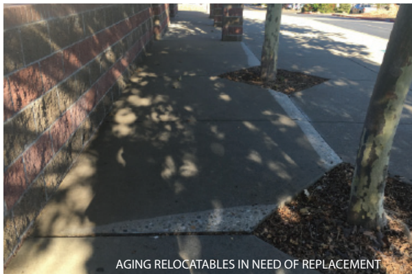
AGING RELOCATABLES IN NEED OF REPLACEMENT
