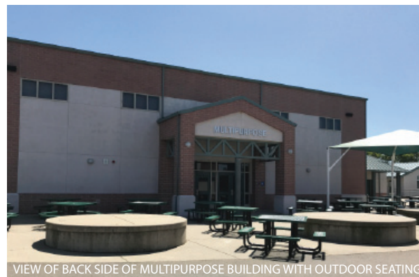
VIEW OF BACK SIDE OF MULTIPURPOSE BUILDING WITH OUTDOOR SEATING
