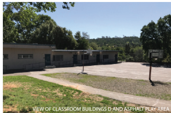
VIEW OF CLASSROOM BUILDINGS D AND ASPHALT PLAY AREA
