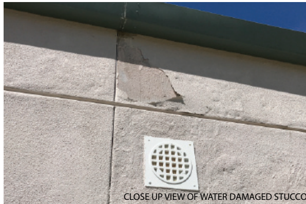
CLOSE UP VIEW OF WATER DAMAGED STUCCO
