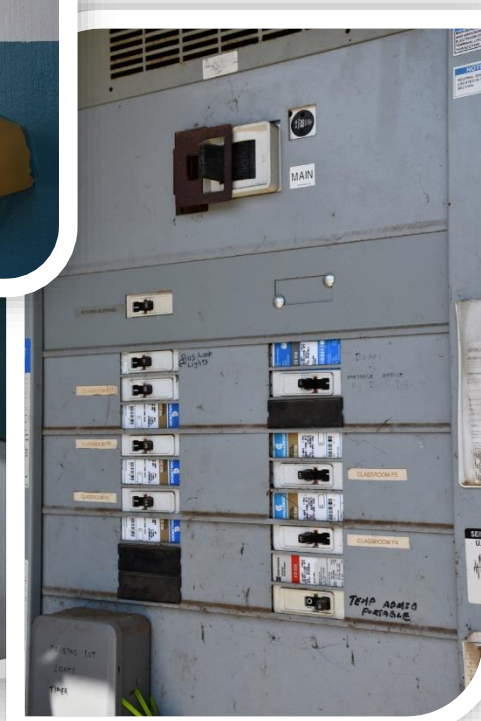
Outdated electrical systems
