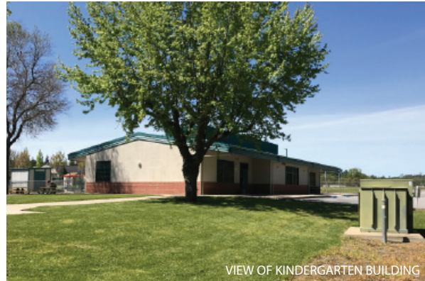
VIEW OF KINDERGARTEN BUILDING
