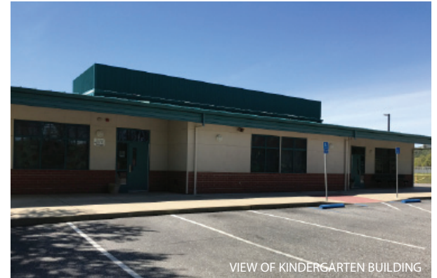
VIEW OF KINDERGARTEN BUILDING
