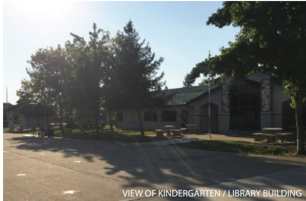
VIEW OF KINDERGARTEN / LIBRARY BUILDING
