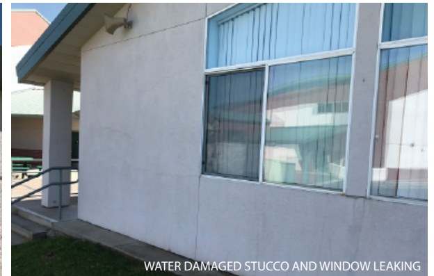
WATER DAMAGED STUCCO AND WINDOW LEAKING
