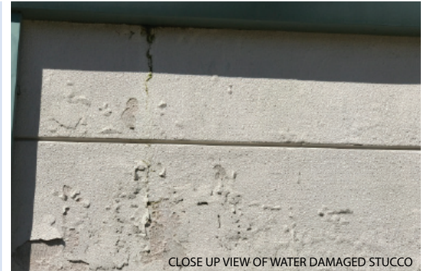
CLOSE UP VIEW OF WATER DAMAGED STUCCO
