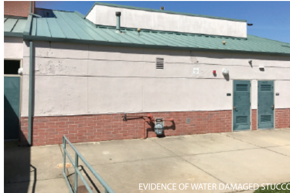
EVIDENCE OF WATER DAMAGED STUCCO
