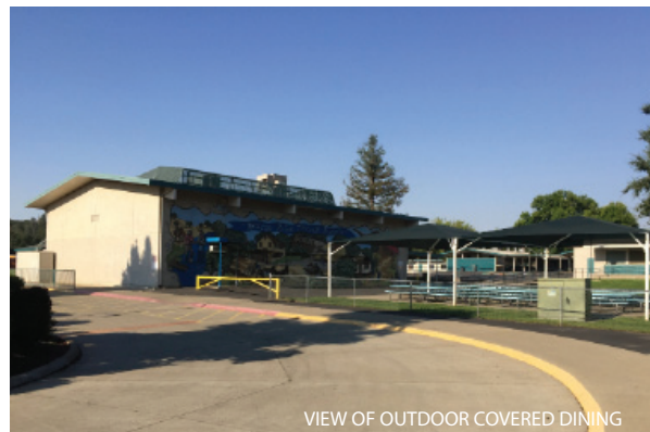
VIEW OF OUTDOOR COVERED DINING
