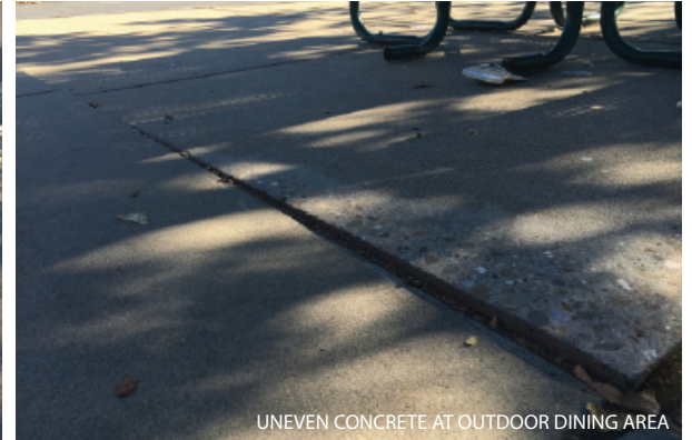
UNEVEN CONCRETE AT OUTDOOR DINING AREA
