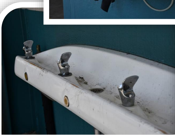
Antiquated facilities and fixtures
