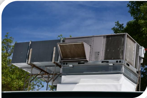
Old HVAC units need to be replaced with energy efficient models
