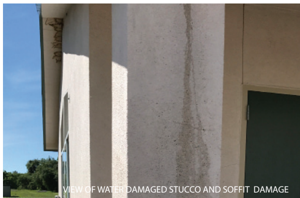
CLOSE UP VIEW OF WATER DAMAGED STUCCO
