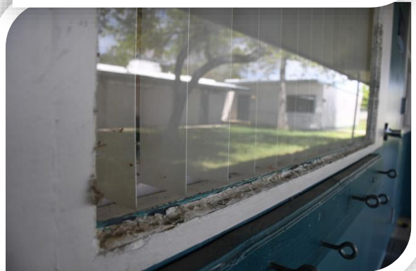
Aging windows must be replaced
