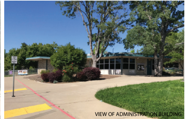
VIEW OF ADMINISTRATION BUILDING
