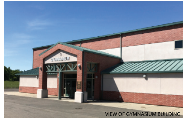
VIEW OF GYMNASIUM BUILDING
