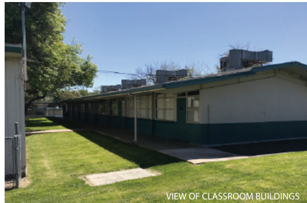
VIEW OF CLASSROOM BUILDINGS
