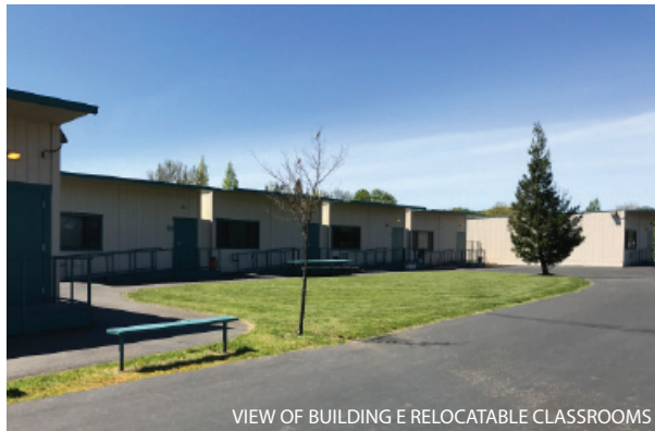
VIEW OF BUILDING E RELOCATABLE CLASSROOMS
