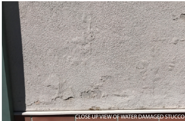
CLOSE UP VIEW OF WATER DAMAGED STUCCO
